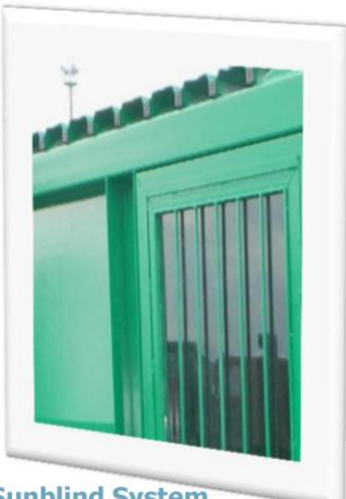
Sunblind System sunblind on the container to protecting from strong solar irradiation
